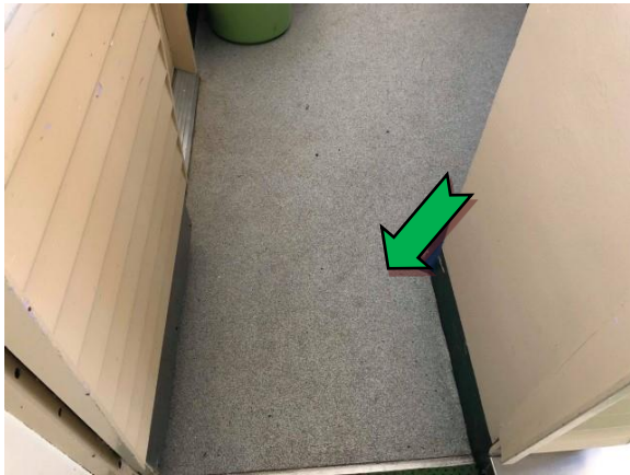
Photo 9. Interior, bar area, floor coverings – suspected non asbestos-containing sheet vinyl.
