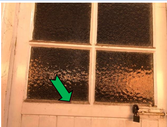
Photo 5. Exterior, east elevation, shed, door – non asbestos-containing window caulking.
