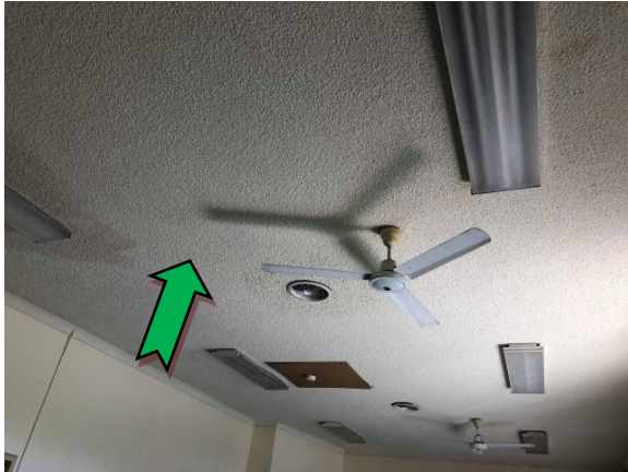
Photo 7. Interior, bar area, ceiling – non asbestos-containing vermiculite.
