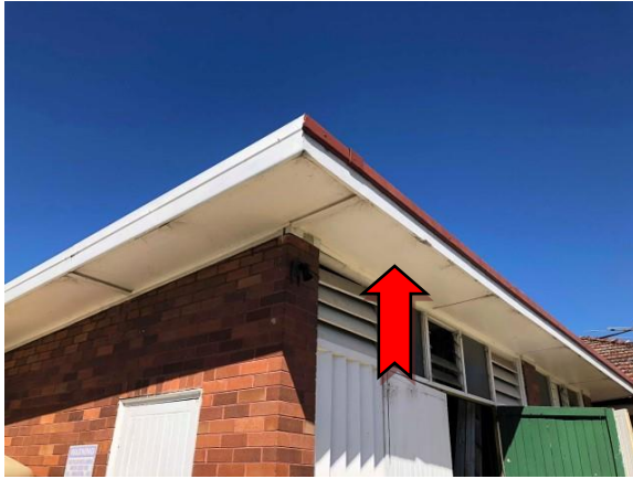
Photo 1. Exterior, eastern elevation, shed, eaves – asbestos-containing fibre cement sheeting.
