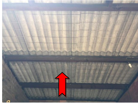
Photo 2. Exterior, eastern elevation, shed, roof – asbestos-containing moulded fibre cement.
